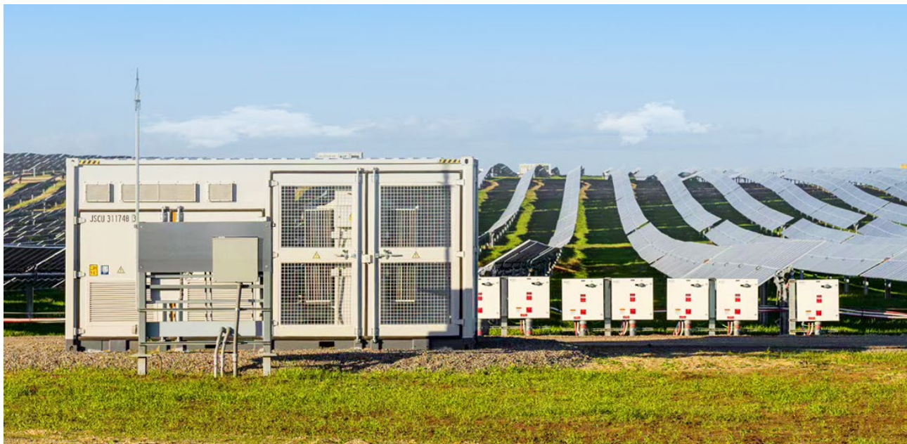
Fig-5: 200MW plant using central inverter + bifacial modules + tracker in California, USA
